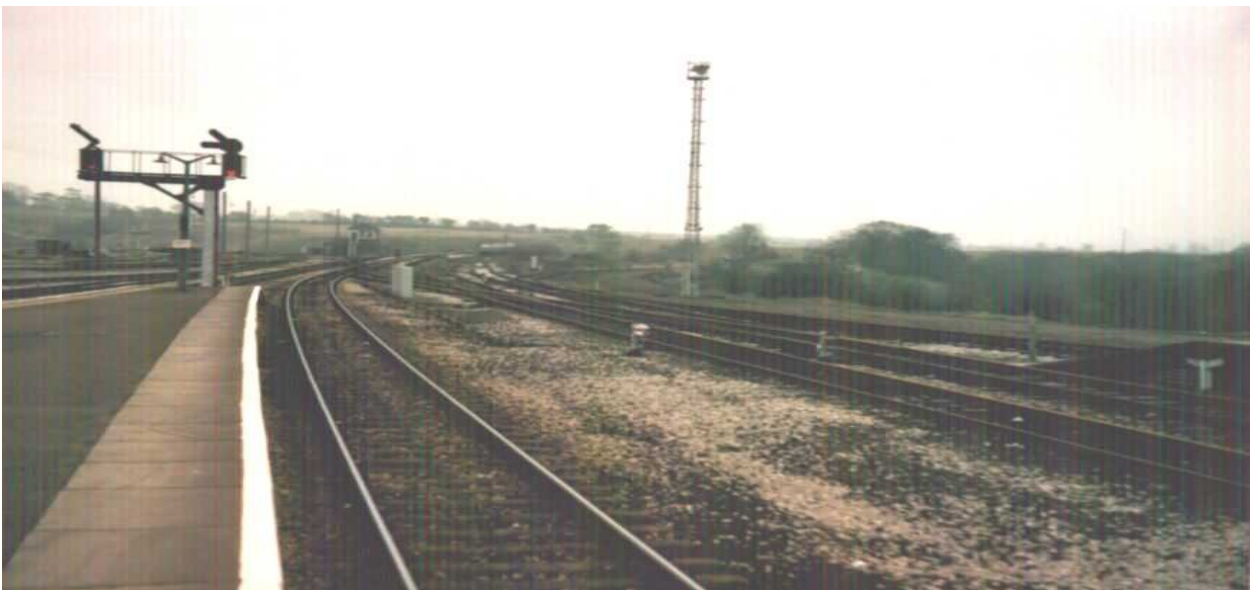
Figure 3.4. The Eastern End of Yeovil Junction Station, The Southern Chord can be seen on the right.
